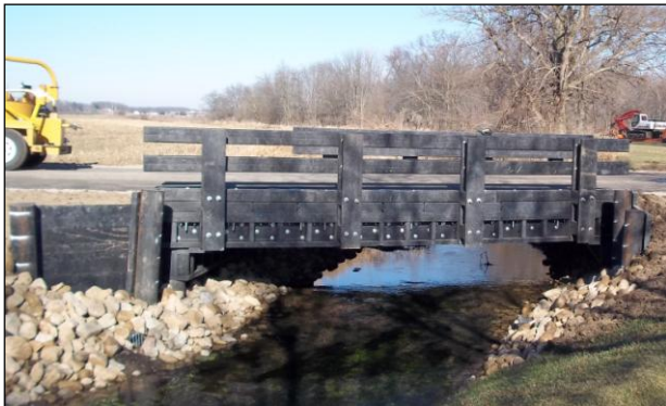
Bridge 174-0.56 over the Onion Ditch
